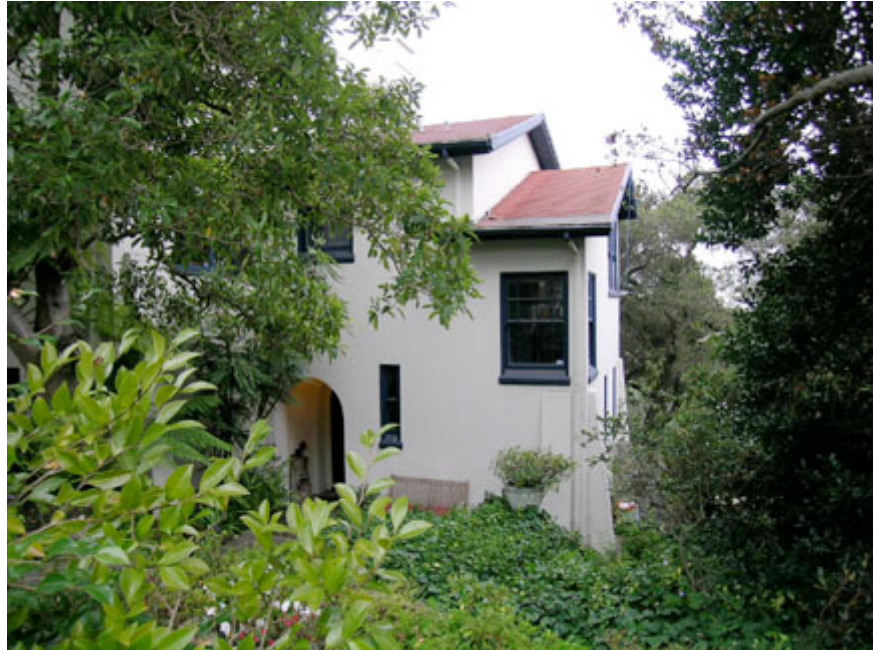
Part of the façade on Thousand Oaks Blvd., formerly Escondido Avenue (photo: Daniella Thompson, 2007)
